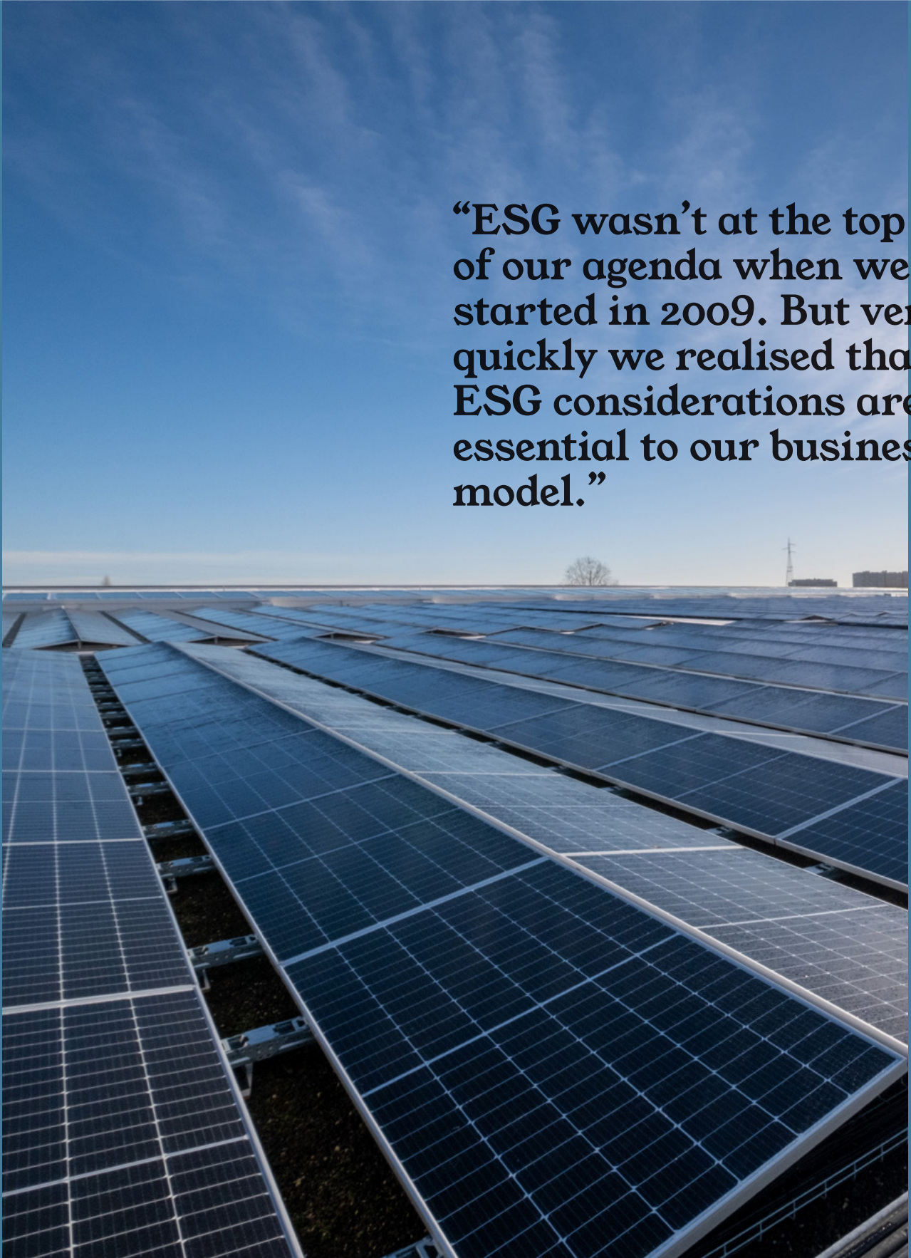
Solar panels on the roof of our new flagship project "Malinas" in Mechelen.
