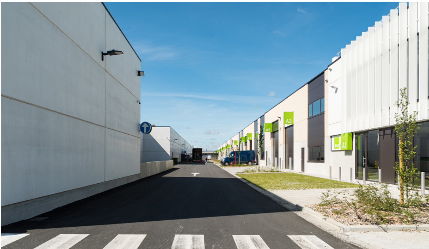
Example of a mixed-use development in Wavre which has a consumer-facing retail park backing onto SME and light industrial units.
